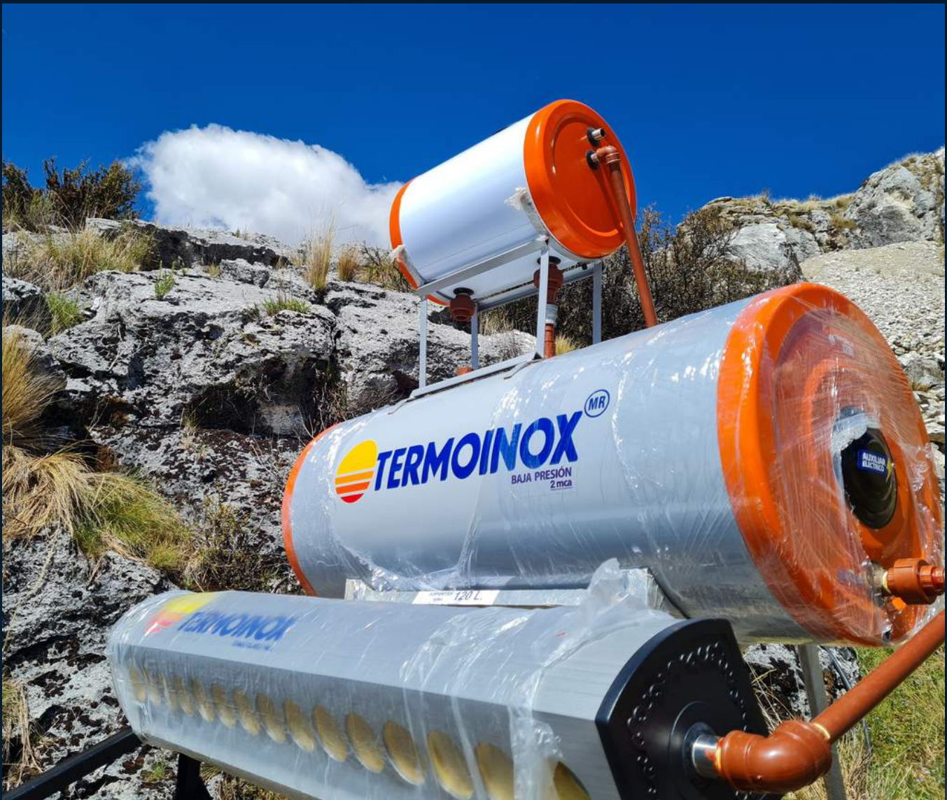
Solar water heaters in process of installation
